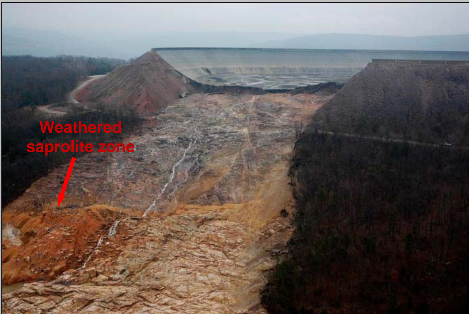
Geologic units exposed by scouring of the outbreak flood. Note the reddish saprolite. Photo from the Associated Press
