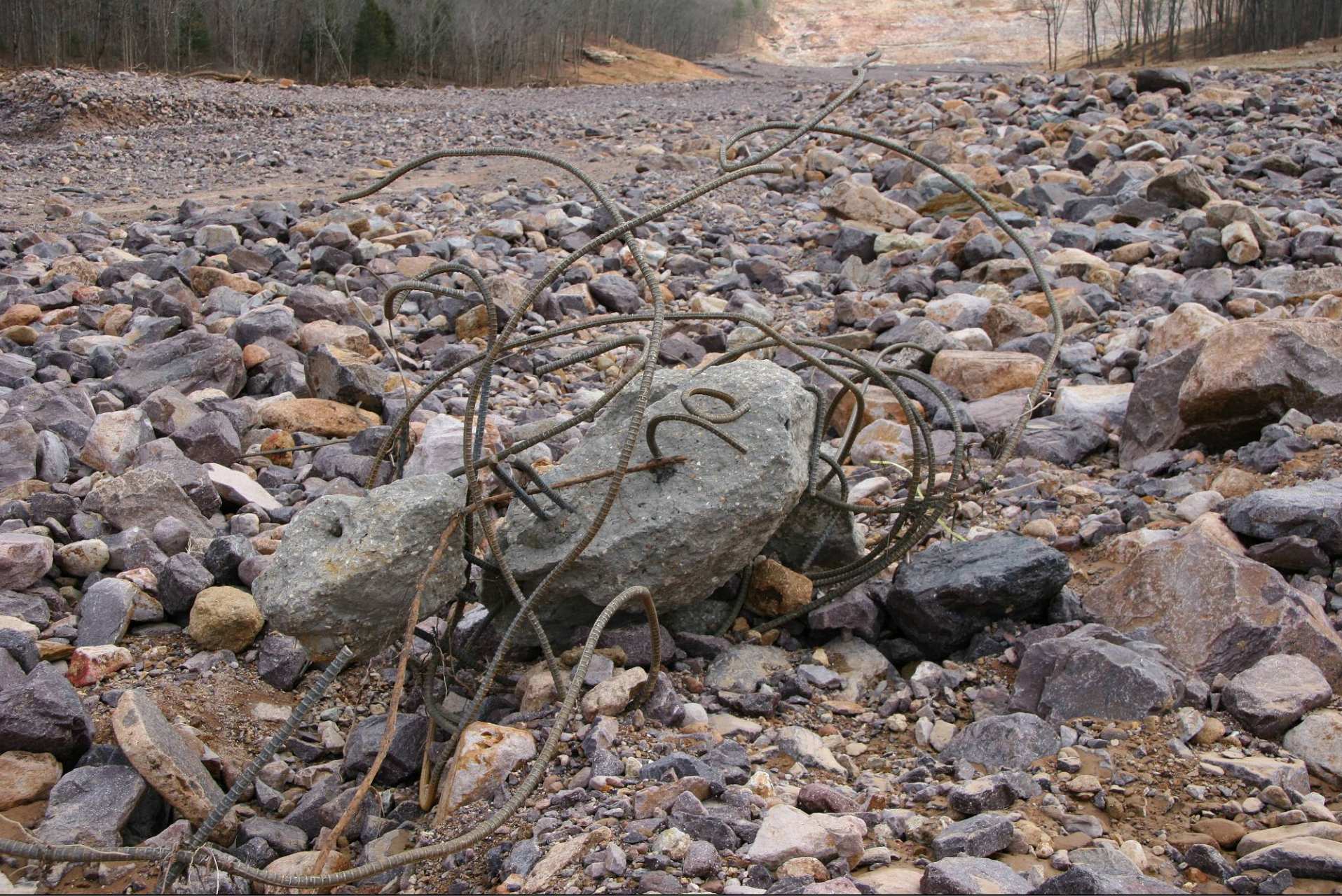
Concrete and rebar from the dam littered the scour channel.
