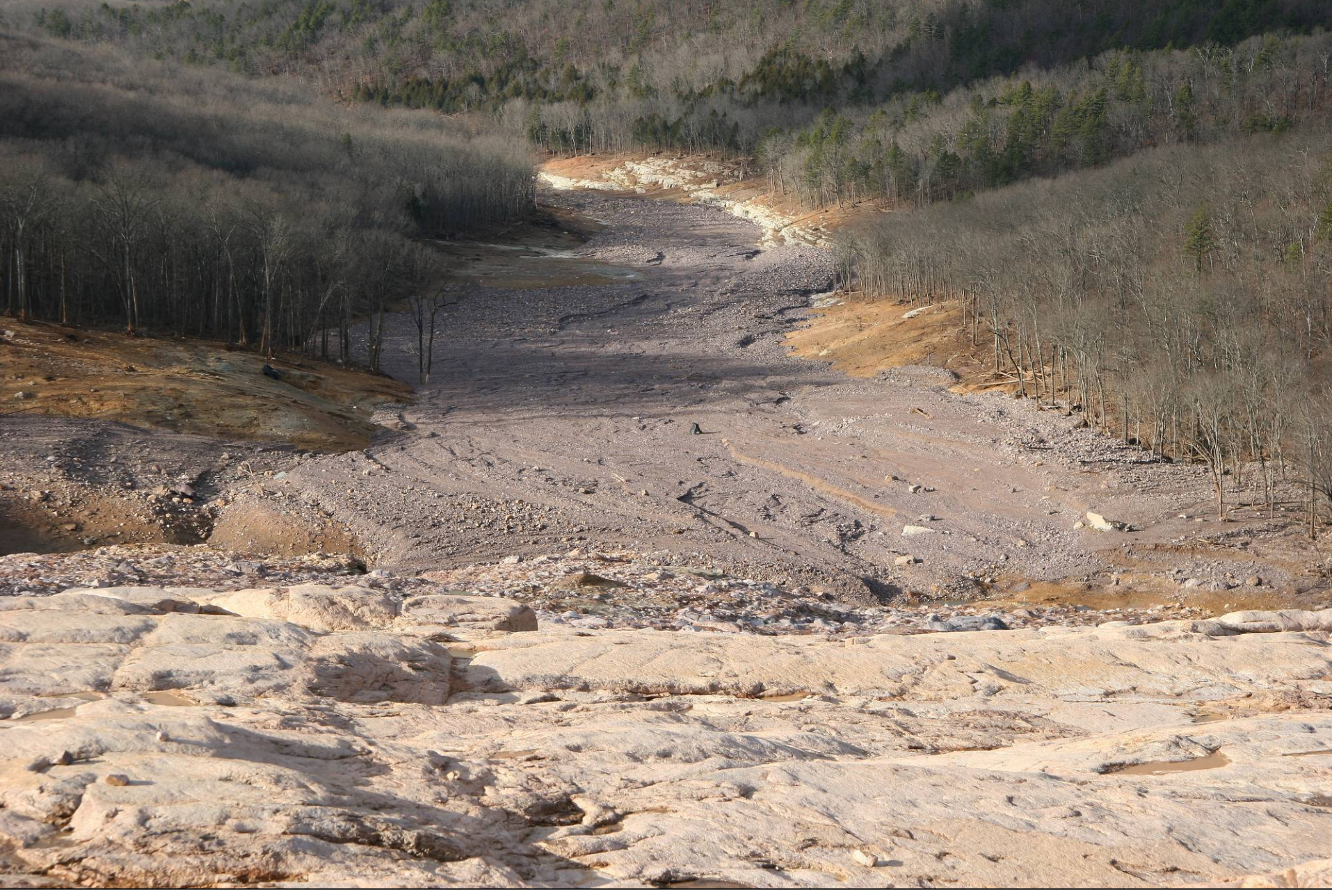
Lower portion of the scour channel and precipitous drop, immediately below the reservoir.
